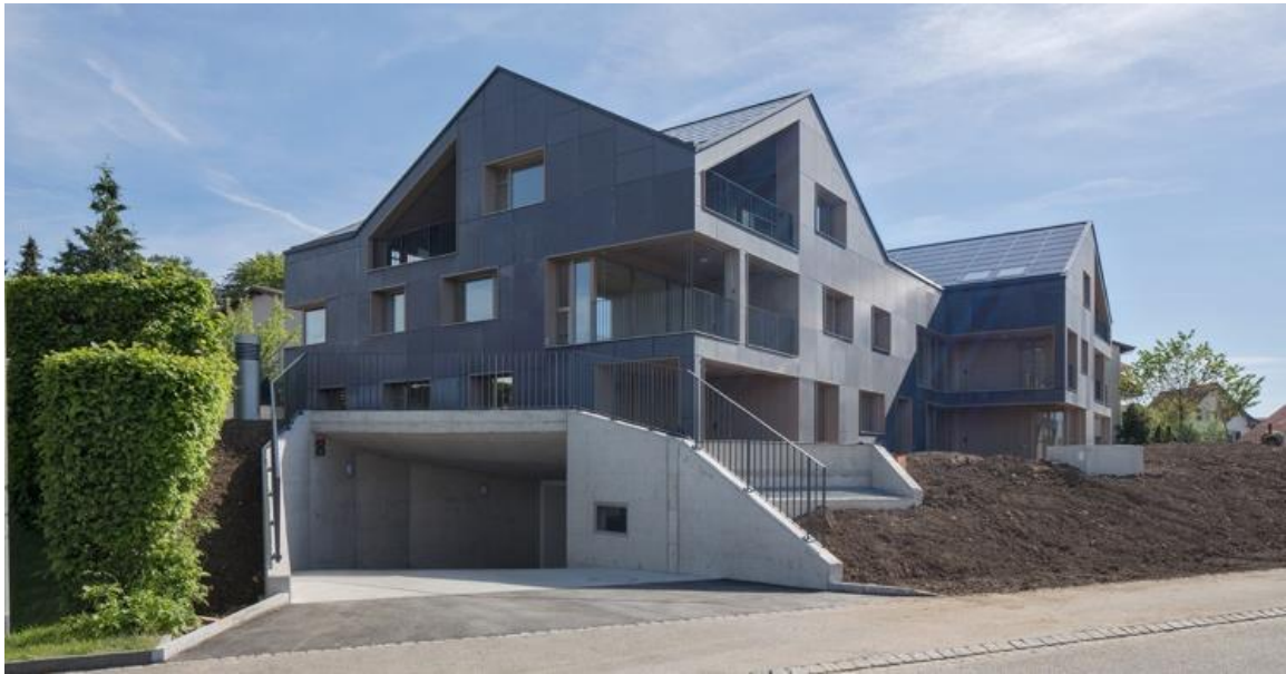
Image 2: Grid-defected multi-family building in Brütten, completed 08/2016 @René Schmid Architekten
